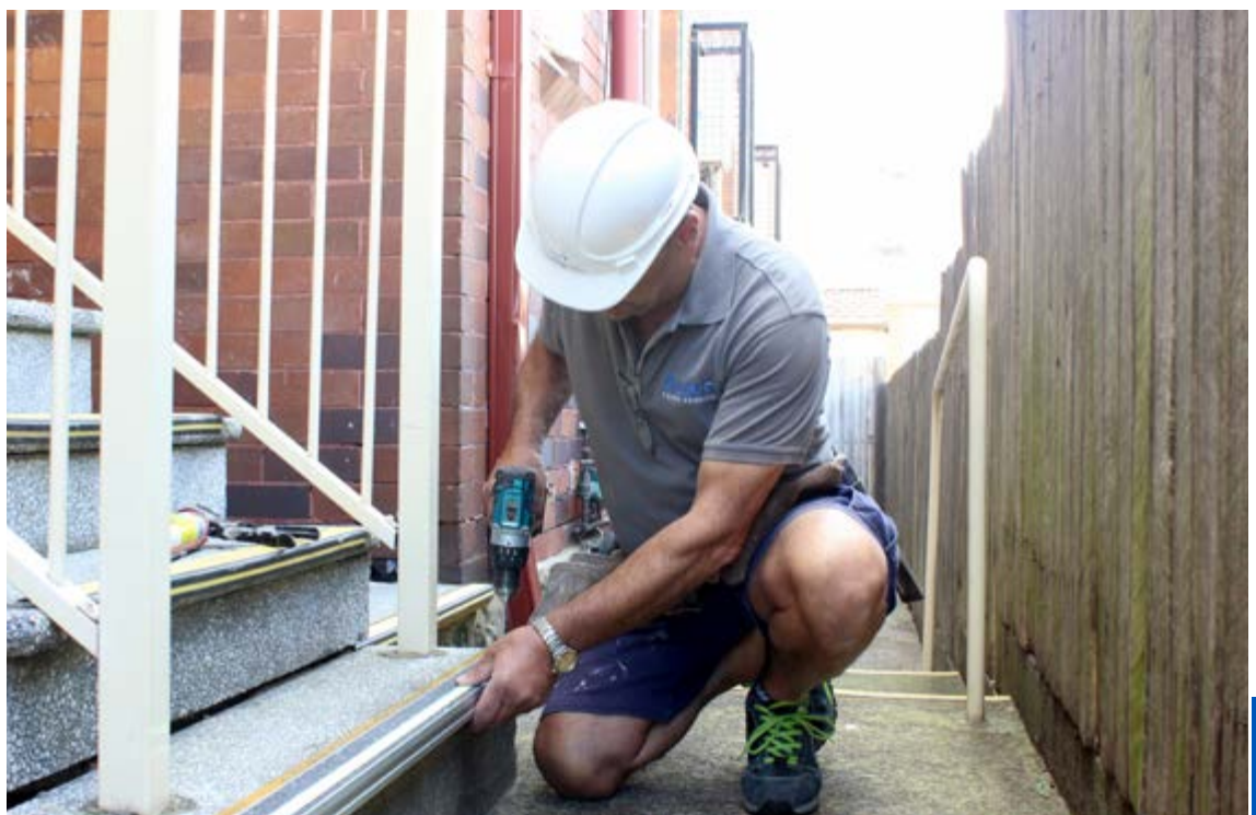
Assett Contractor fitting non-slip strips to external steps
